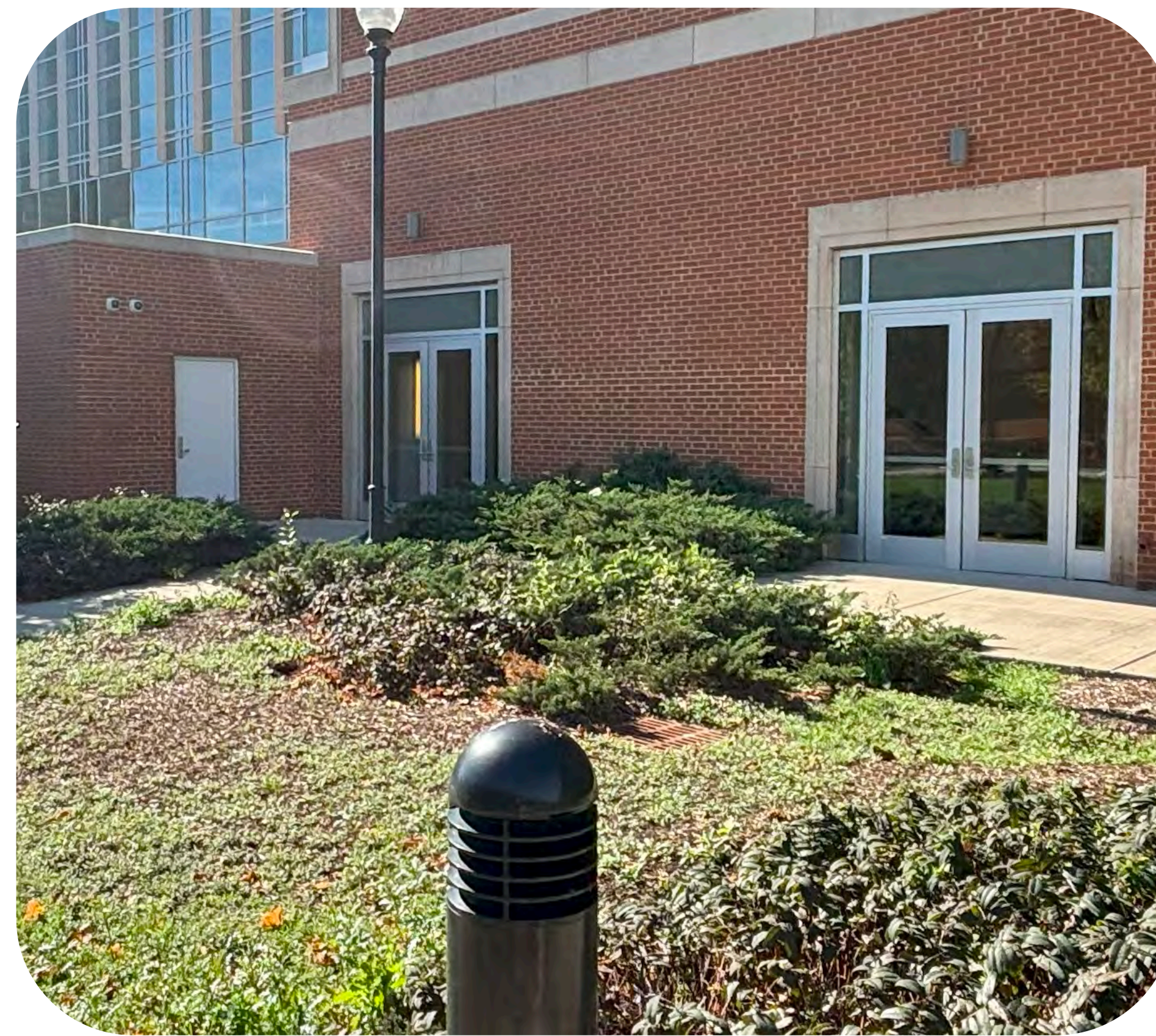
Lower Level Entrances
