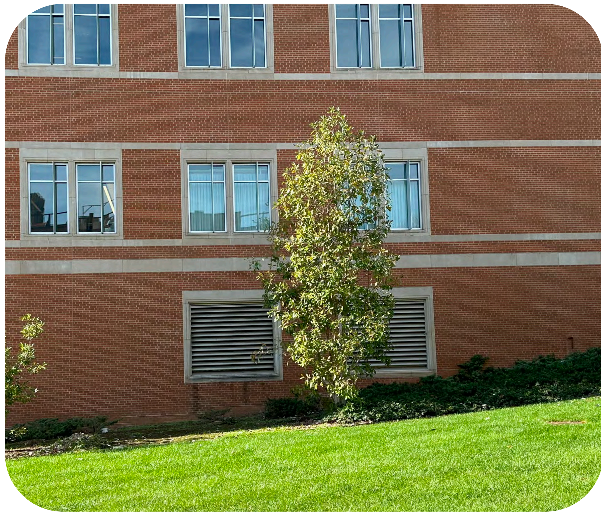
Air Intake Vents (approx. 898 elevation)
