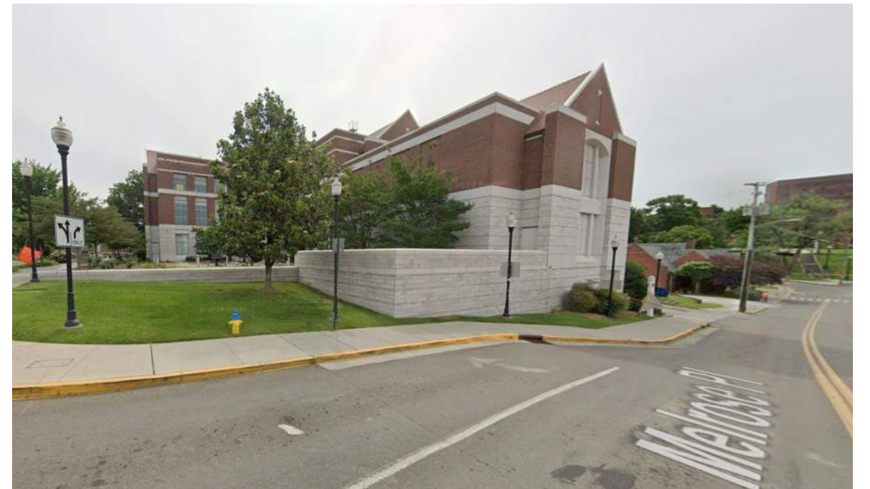
View of Northwest Corner
