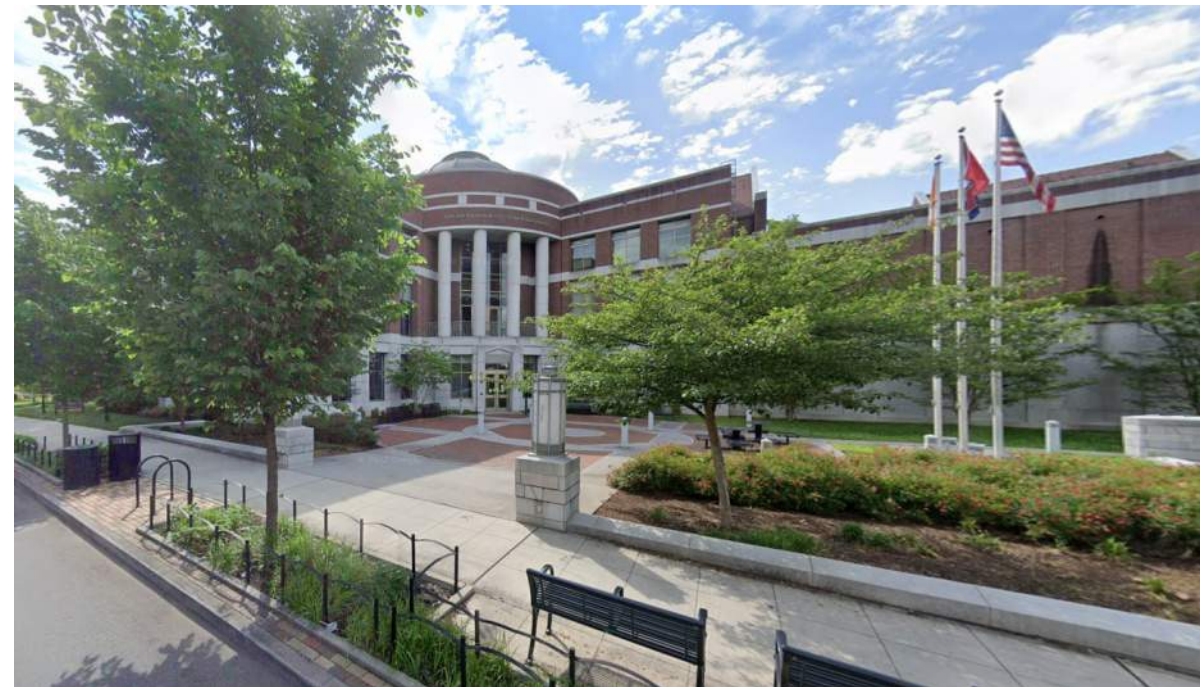
View of entry and North Elevation
