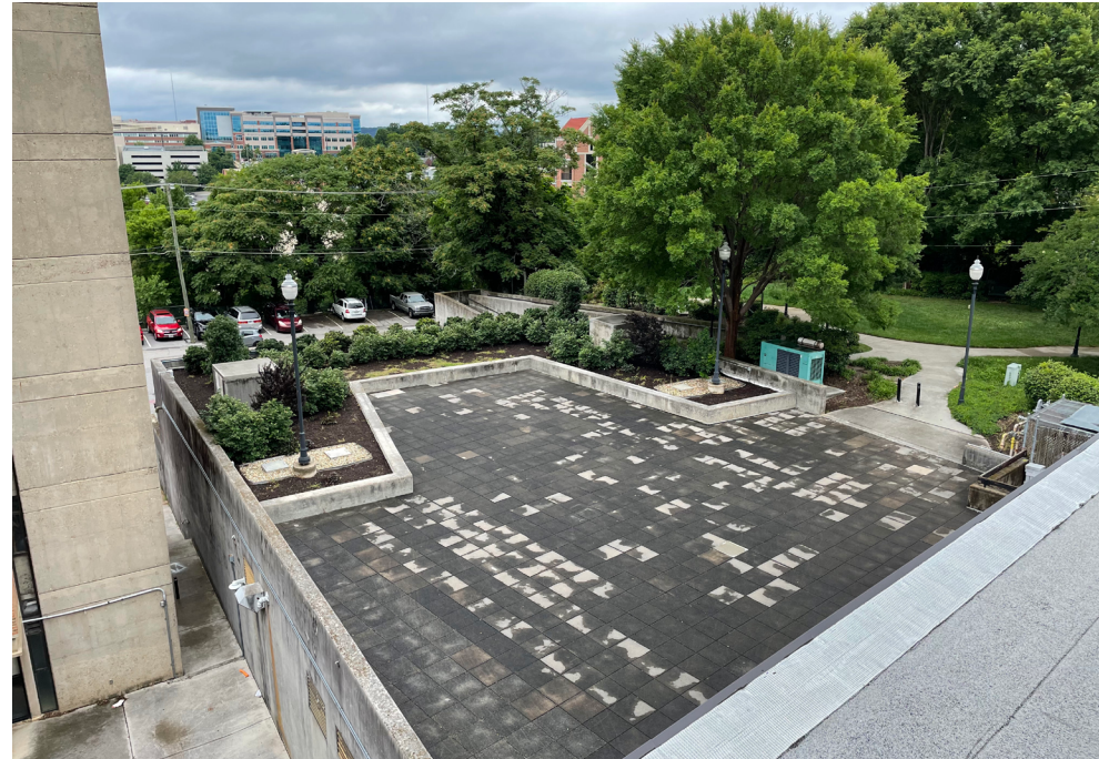
(above) Existing occupiable roof over portion of Basement Level.
