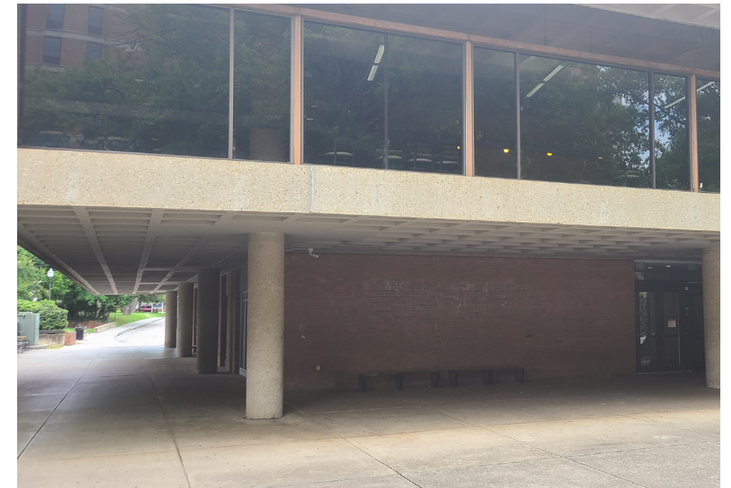
(above) Existing exterior glass wall system at Second Level.
