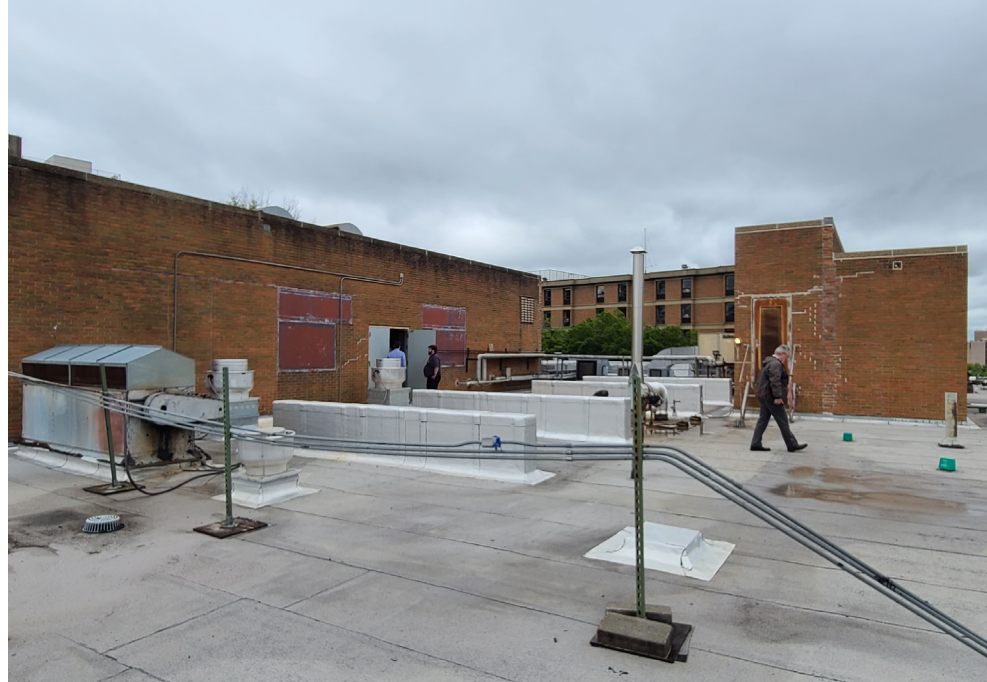
(above) Existing Roof; view towards Mechanical Penthouse.
