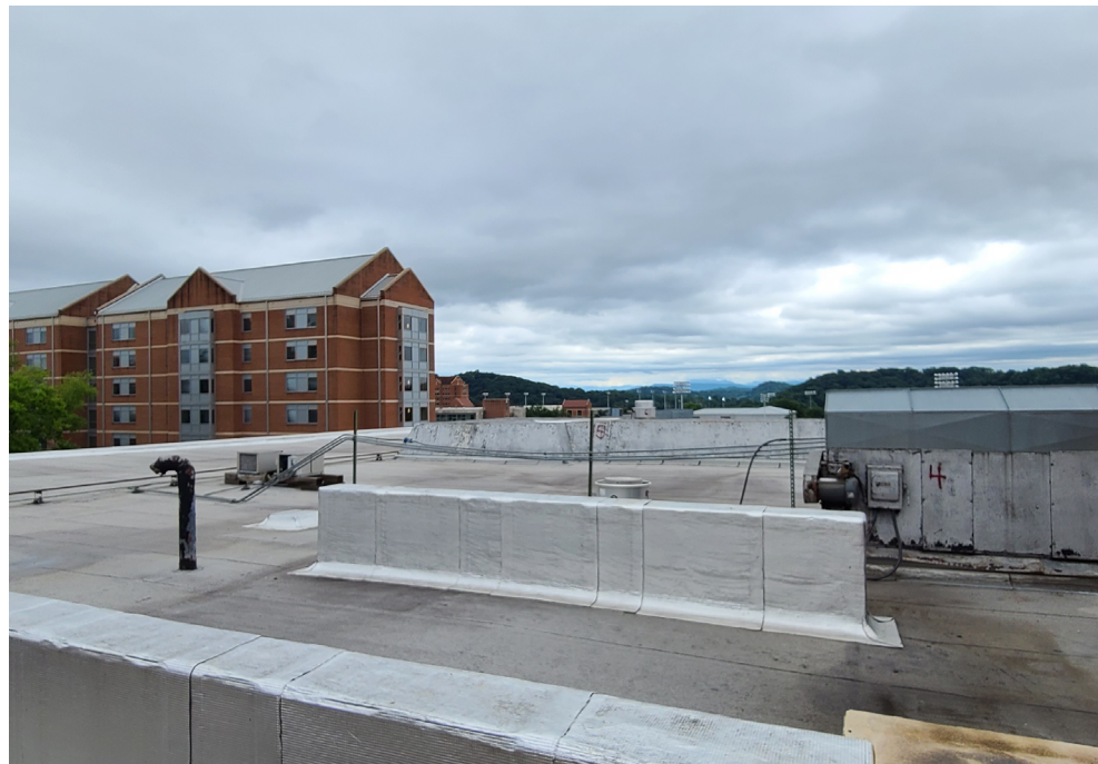
(above) Existing Roof
