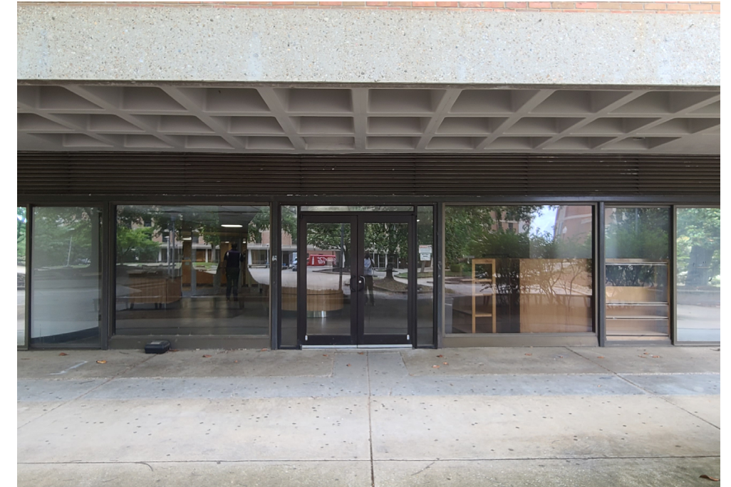
(above) Existing exterior glass entrance system.
