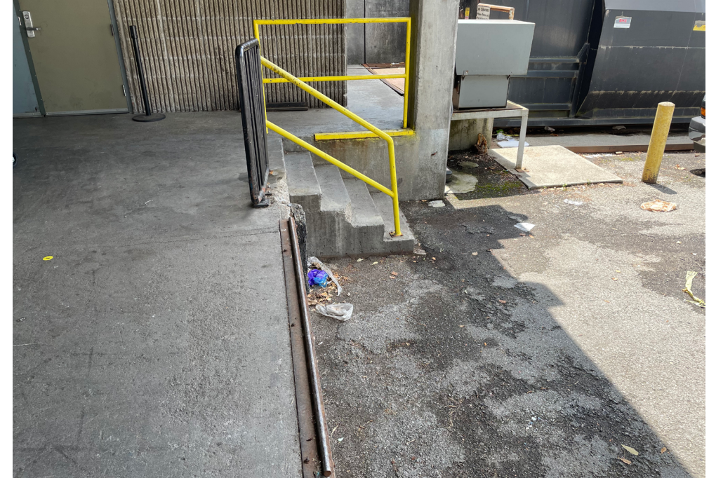
(above) Existing Loading Dock
