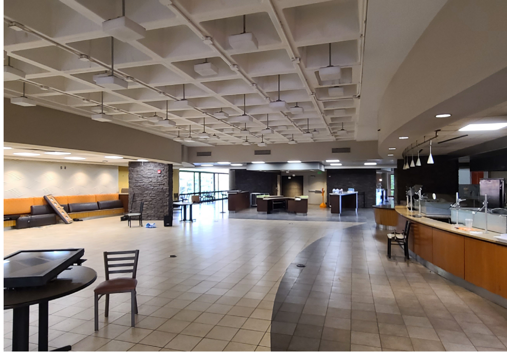
(above) Existing Dining Space; view of exposed waffle slab.
