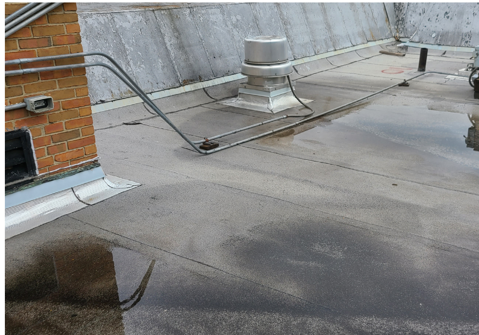
(above) Existing Roof; view of pooling water.
