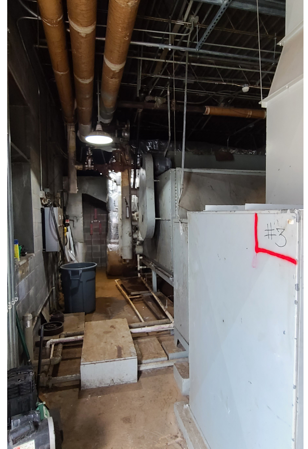
(above) View of interior of existing Mechanical Penthouse.
