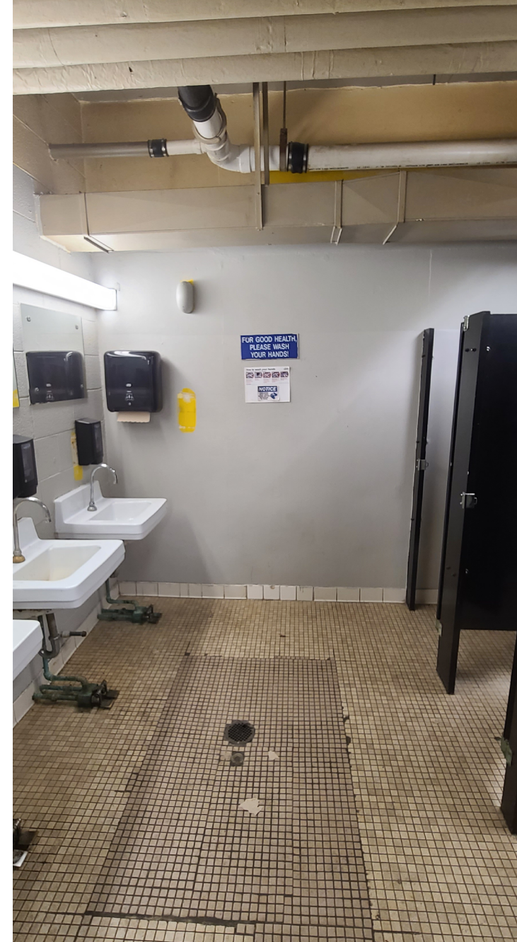
(above) Existing Restrooms
