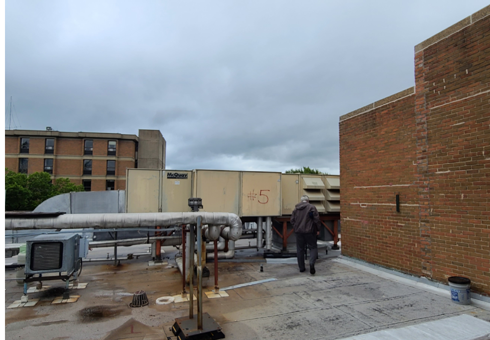
(above) Existing Roof; view of rooftop units and ductwork.
