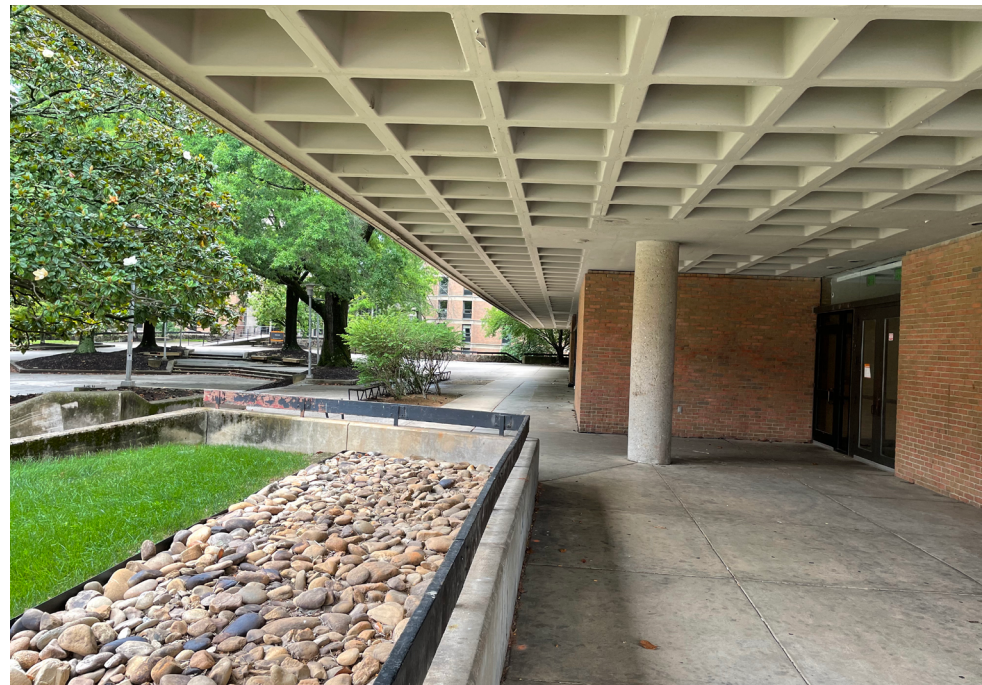
(above) Existing exterior; view of existing waffle slab and adjacent existing planter and railing.
