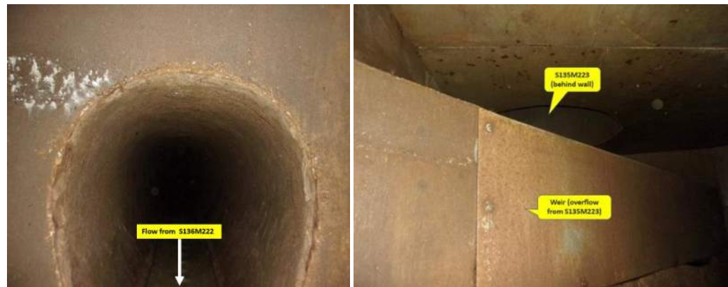
Figure 2.1.1.2. Incoming egg-shaped sewer and weir wall in Mabel St Regulator (S135M223)
